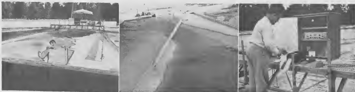
A MOVABLE bridge, left photo, was installed for measuring purposes. The bridge rolls on UN BRUG mobil, foto robes, a wórdé instala pa obhetionan di registracion. E brug ta kora two elevated rails, one on the "tree" and one on the "mainland." At the west entrance of the aruba den haaf, foto drechi, ta un dam móbil. Banda drechi ta e registrador di ola.
